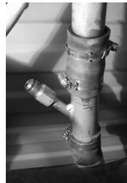
Figure 7: Installing 'Return to Tank' assembly
